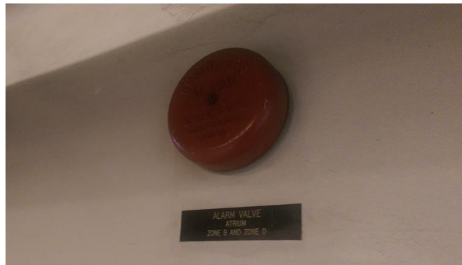
Figure 11 : Fire alarm bell
