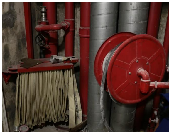
Figure 20: Wet riser
