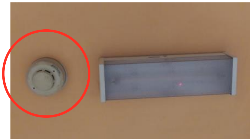
Figure 2 : Photoelectric smoke detector found in San Andreas Mall
