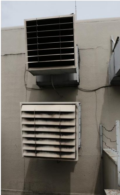
Figure 3.1: Extract system located on the roof top drawing out the dirty air from the basement
