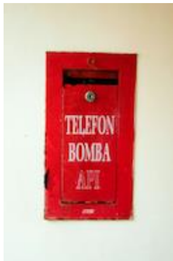
Figure 8 : Fireman intercom system remote handsets
