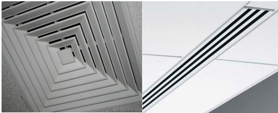
Square diffuser (right) and linear diffuser (left)
