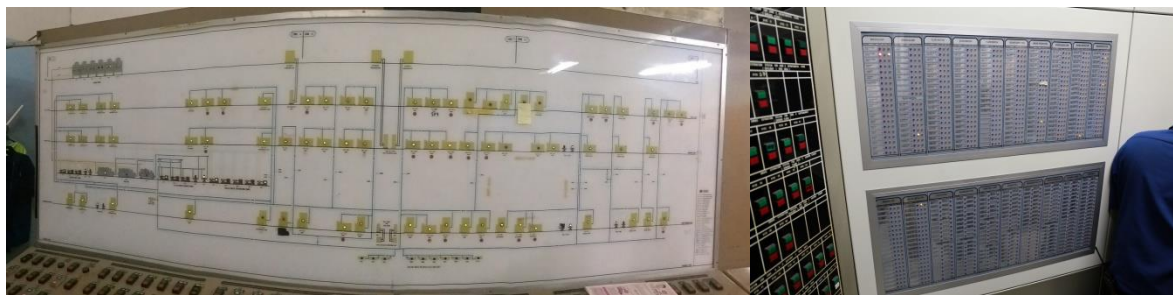
Figure 4 : transmission of fire signals through fire control panel
