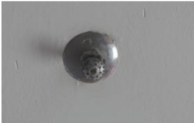
Figure 13 : Pendent sprinkler
