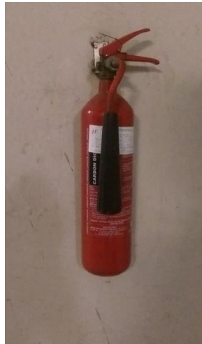
Figure 24: Carbon dioxide fire extinguisher
