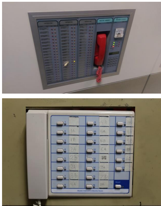
Figure 9 : Emergency and EWIS at the fire control room
