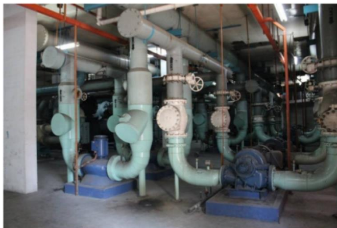
Condenser water pumps
