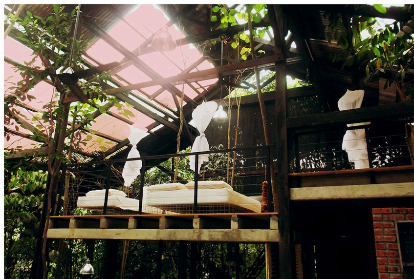
Figure 4.5: Transparent roof panels to allow sunlight into the building.
