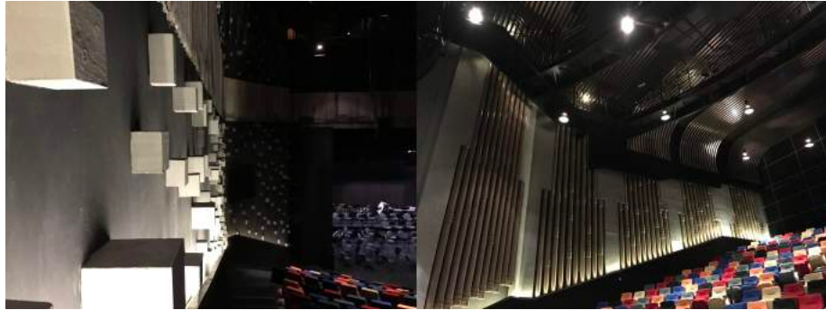
Figure 3.19: Sound diffusers can be seen on the both sides of the walls of Pentas 1, KLPAC by using DIY items such as PVC pipes and white boxes.
